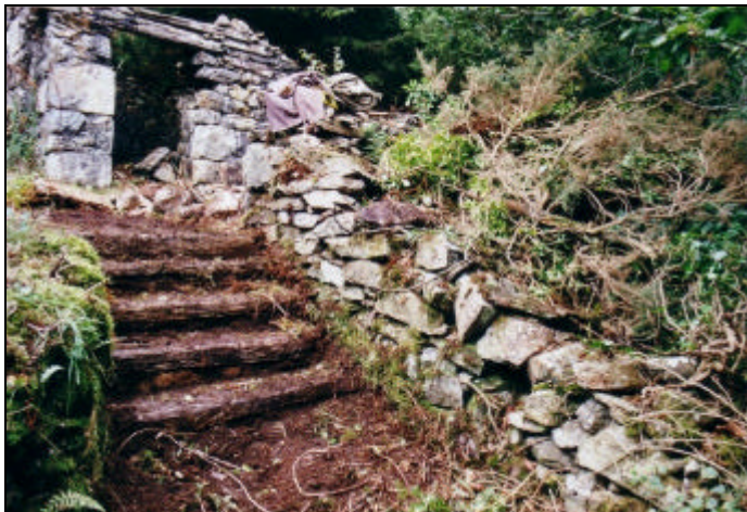
One of the sets of steps revealed at the Smithy
